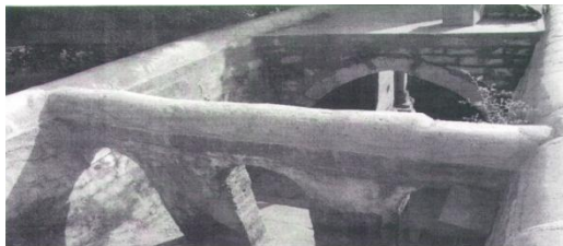
Inner steps of Dhoriwav on Junagadh Road
